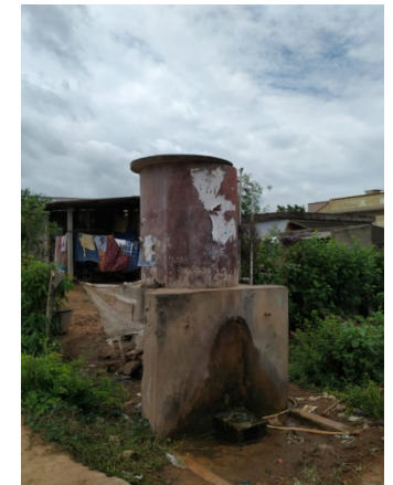
Figure 5.11: Condition of Water supply
