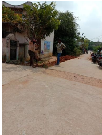
Figure 5.8: Condition of Roads
