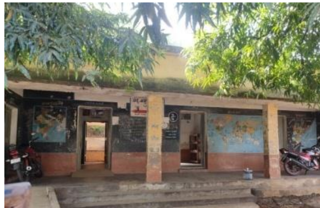
Figure 4.7: Condition of village school
